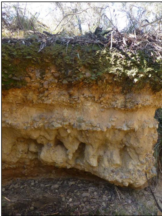
Fig. 7. An erosion gully low in the footslope revealing several different layers of alluvial deposits—well-rounded stone, gravels and soils. Note that this exposure is due to a poorly designed culvert pipe which directs high speed water flow directly onto this drainage line wall. Similar walls close by are not eroding and are covered in cyanobacteria. Photo: R Purdie.
