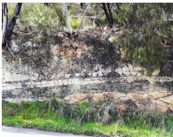
Site 11. About half way up the road to the summit you will find a car park on the left-hand side of a sharp bend in the road. The road cutting opposite the car park area is the geological type section for the Black Mountain Sandstone. (GDA Easting 0690 782 Northing 6093 750)
