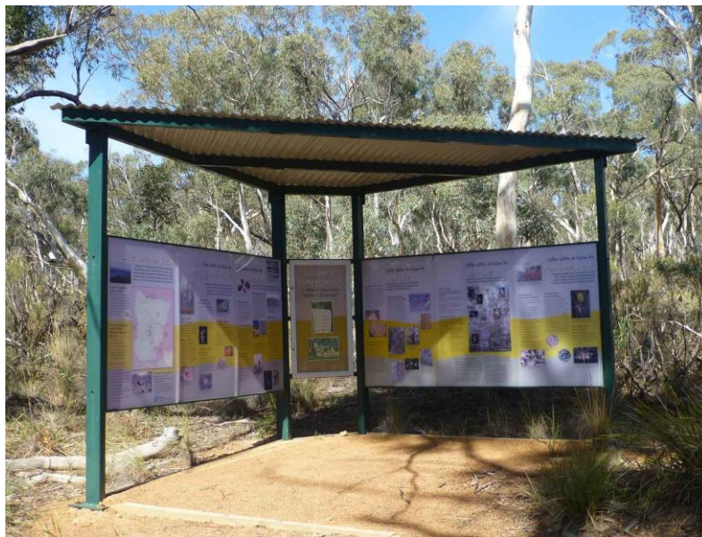
Fig. 6. Canberra Connect sign/shelter on the Link Fire Trail, March 2018. Photo: R Purdie.
