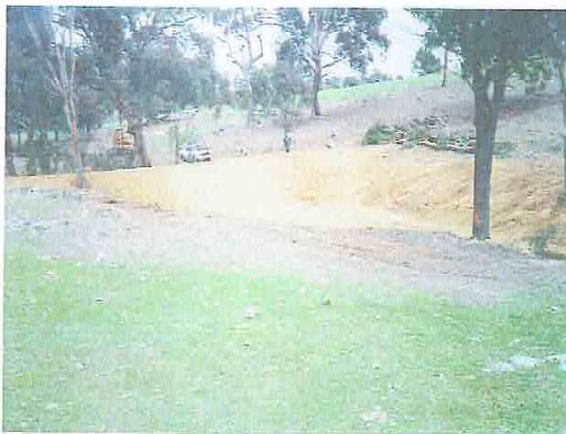
New Dam Construction
