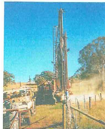
Water Bore Drilling
