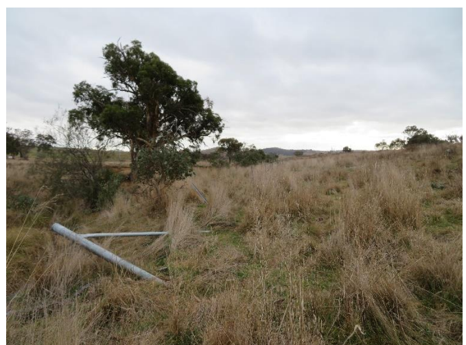
damaged flood gate post
